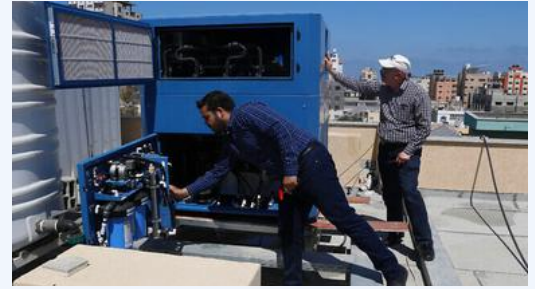
Atmospheric Water Generators (AWG) in Gaza See article
